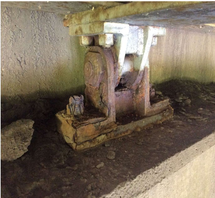
PHOTO 3 Description Bent 1 Bearing 3 (corrosion)
