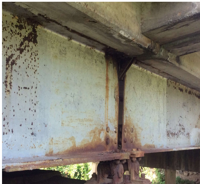
PHOTO 1 Description Girder 1 left @ Bent 3 (corrosion)
