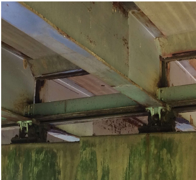
PHOTO 4 Description Girders 2-3 @ Bent 2 (corrosion)
