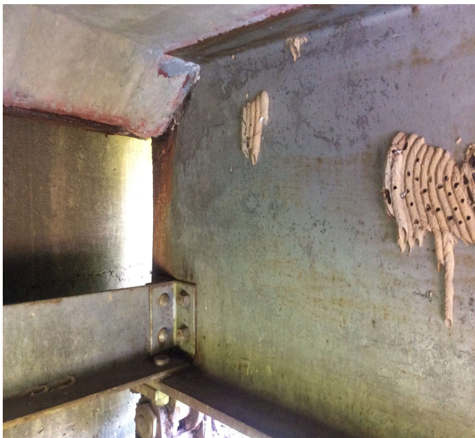
PHOTO 3 Description Span 1 Girder 1 right @ Bent 1 (corrosion)
