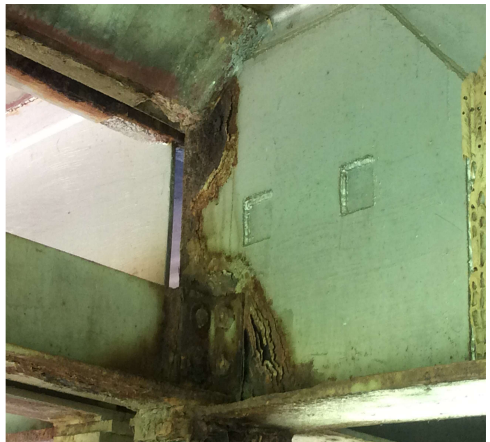
PHOTO 2 Description Span 3 Girder 4 right (corrosion)
