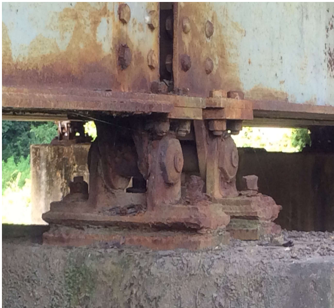
PHOTO 1 Description Bent 3 Bearings 1A & 1B (corrosion)
