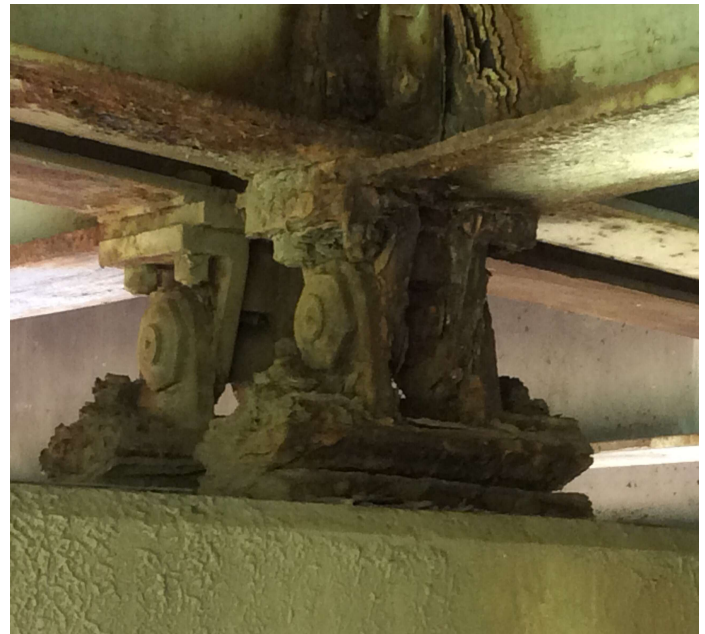
PHOTO 2 Description Bearings 4A & 4B @ Bent 3 (corrosion)
